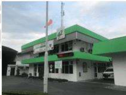
Gambar 2. 1 Gedung Quality Control PT. Petrokimia Kayaku
