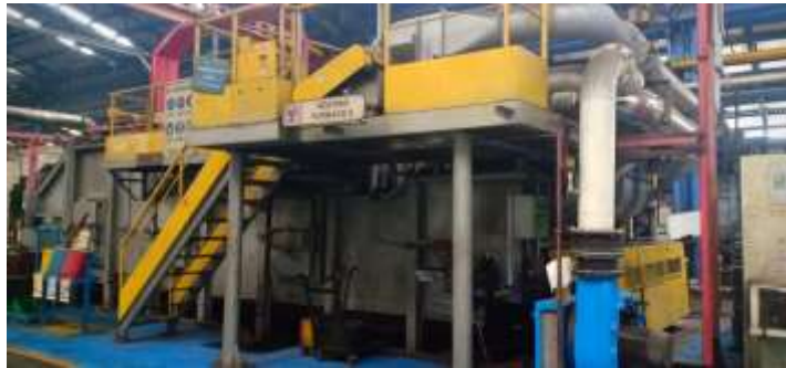
Gambar 2.1 Mesin Heating Furnace
