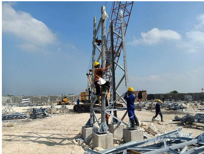
Gambar 7. Rangka Steel Structure 2
