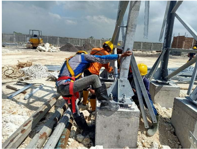
Gambar 6. Rangka Steel Structure
