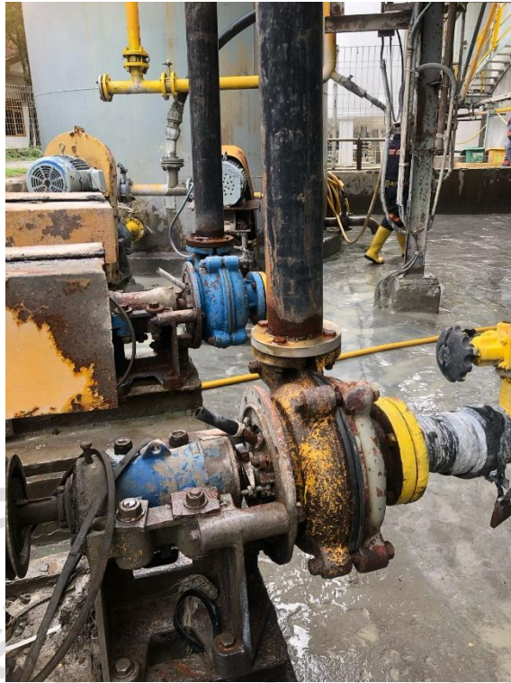
Gambar 4 Pompa Warman Tipe 4/3 EE-HH Filling
