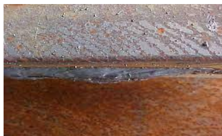
Gambar 2 Defect Gas Hole
