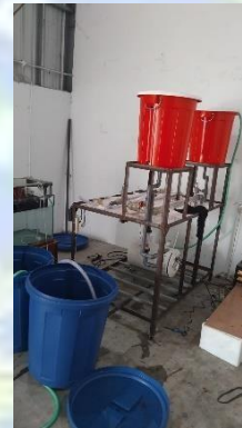
Lampiran 4 Pemasangan water heater
