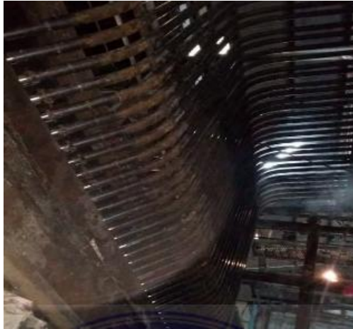
Gambar 2. 4 Pipa superheater sumber (HASIBUAN J., 2023)
