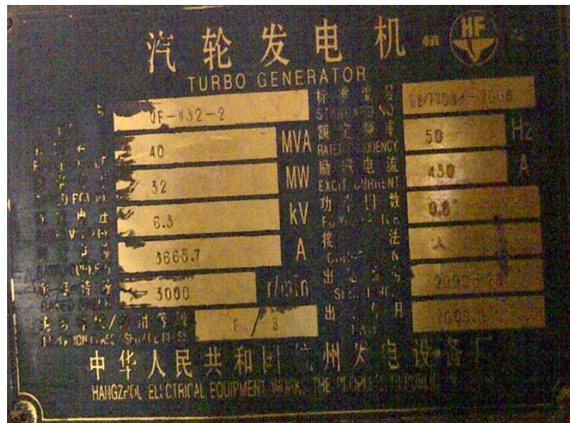
Gambar 3.3 Nameplate Generator PLTU
