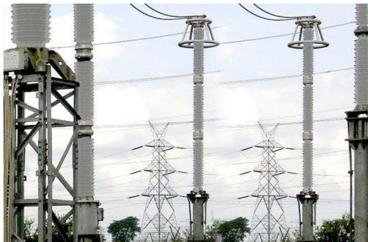
**Gambar 2.23** Lightning Arrester
