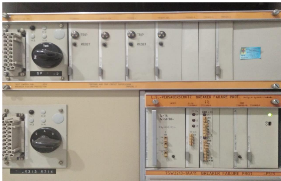
Gambar 2.9. Breaker Failure Protection
