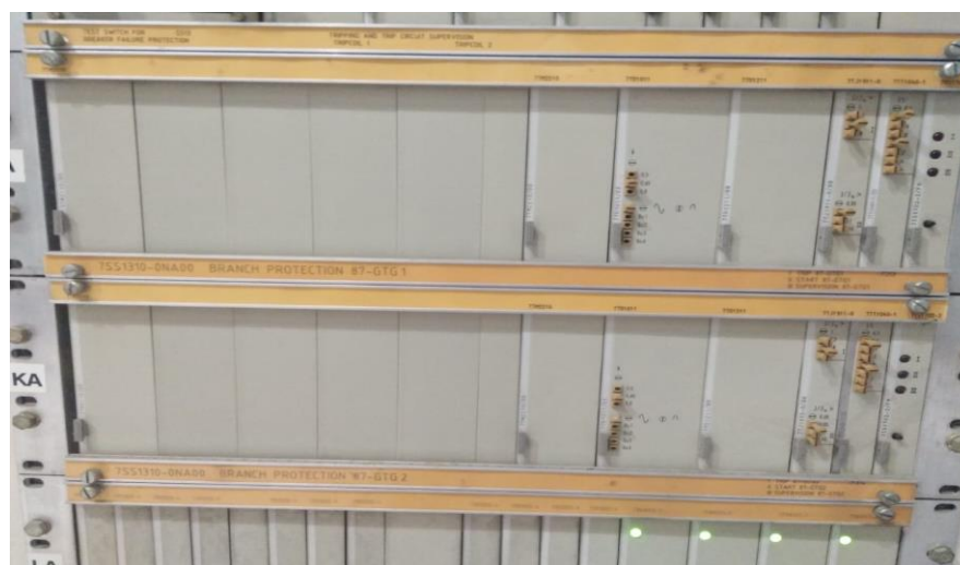
Gambar 2.10. Branch Breaker Failure
