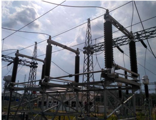
Gambar 2.9 Disconnecting Switch (DS)
