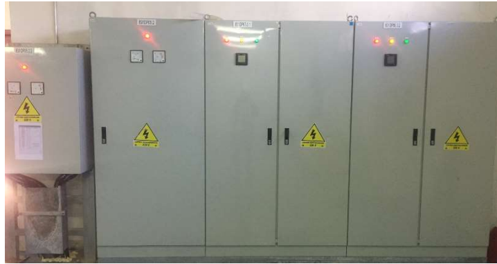
Gambar 2.19 Lighting Distribution Panel
