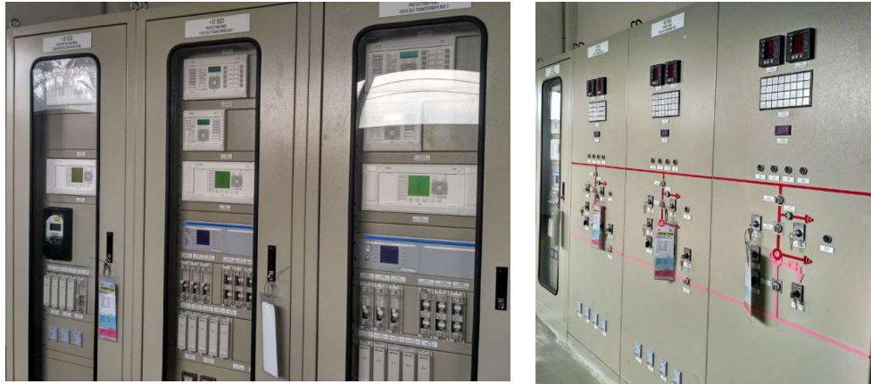
Gambar 2.13 HV Control and Protection Panel
