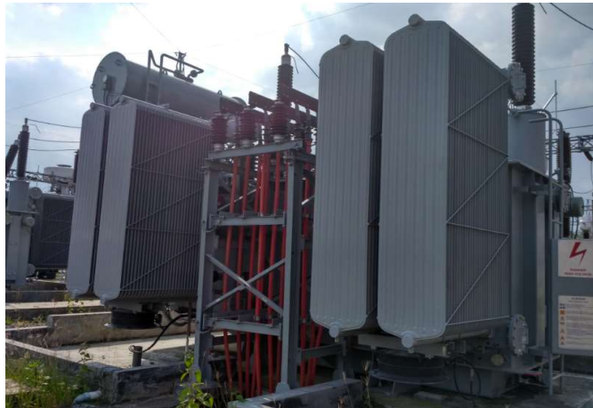
Gambar 2.6 Power Transformer Mainsubstation
