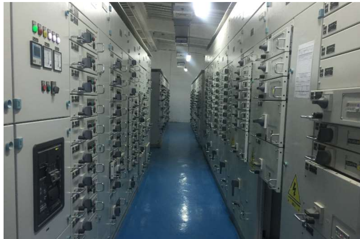
Gambar 2.18 Low Voltage Switchgear & MCC
