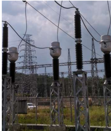
Gambar 2.11 HV Voltage Transformer
