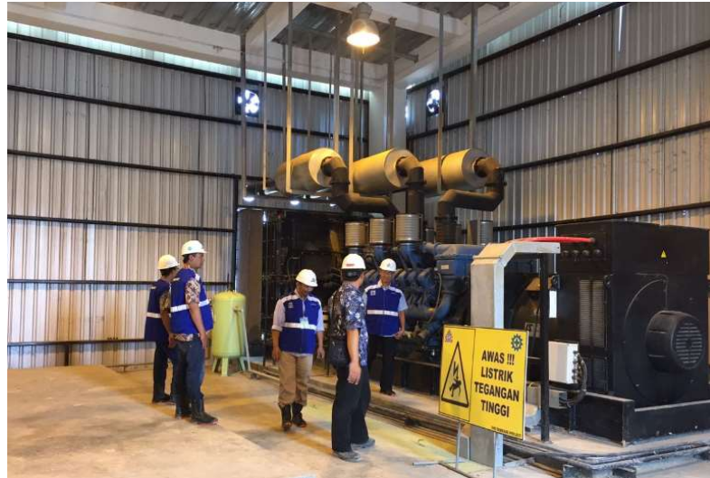
Gambar 2.14 Main Emergency Power 3150 kVA
