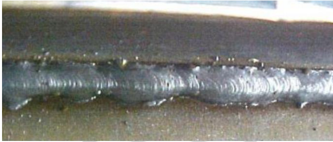
Gambar 4. 3 Defect Las Incomplete Fusion
